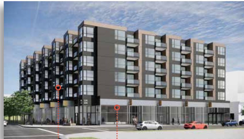
WEST ELEVATION HAS BEEN STEPPED BACK BY 1.5M INTERVALS TO ALIGN WITH PROPERTY LINE PODIUM HAS BEEN VISUALLY SEPERATED FROM THE REST OF THE MASS WITH USE OF MATERIAL
